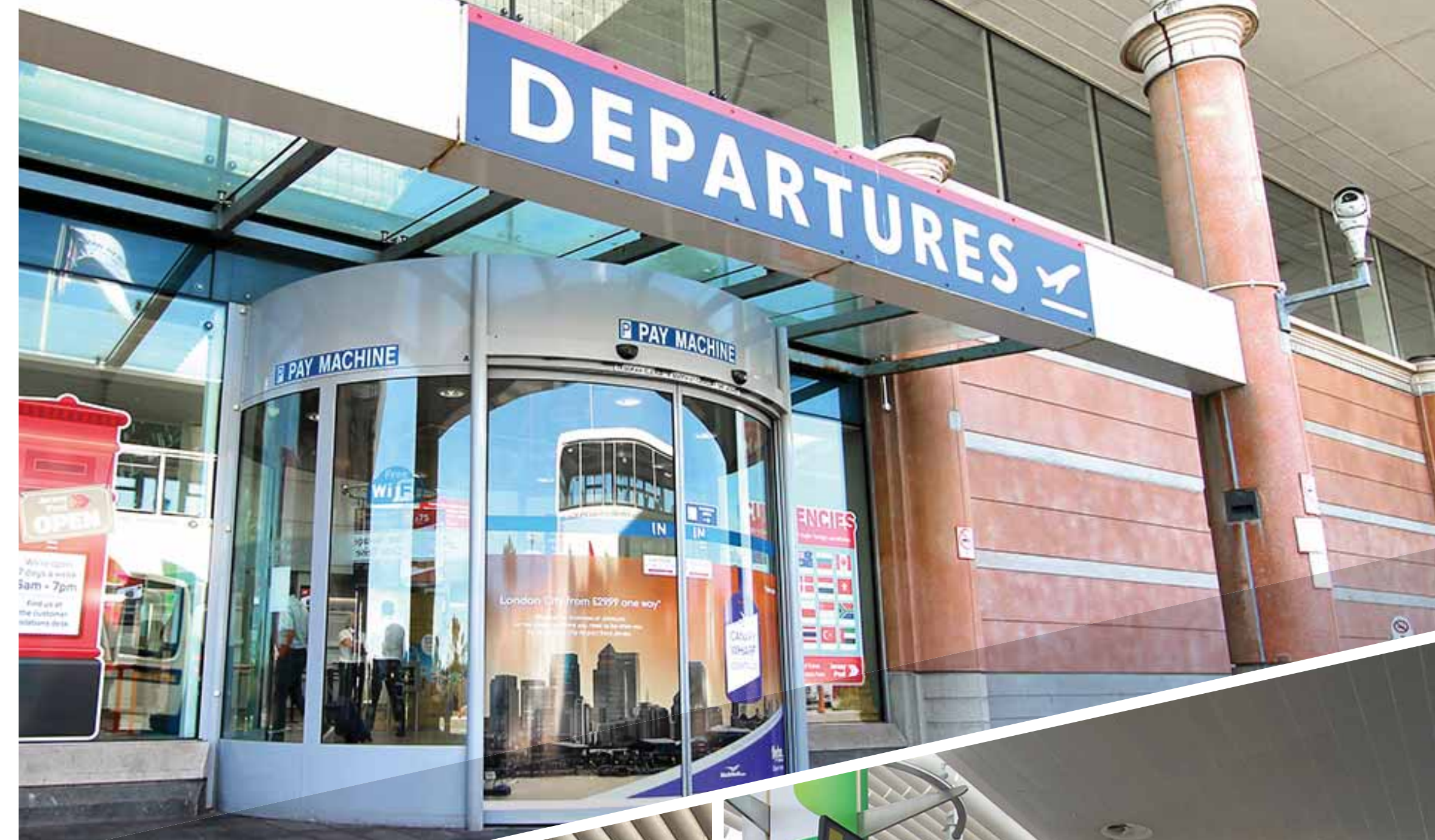
Double-sided Entrance Doors
